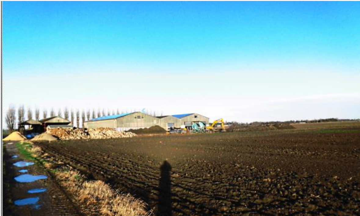
View from the east of Viner station looking west back towards the buildings
