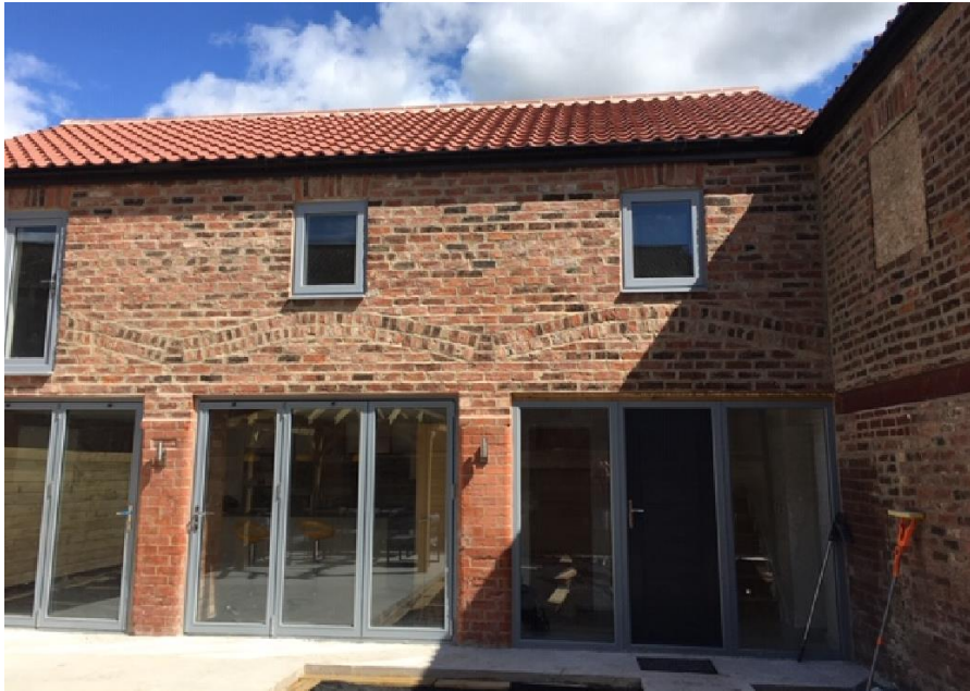
View of the south and west elevations
