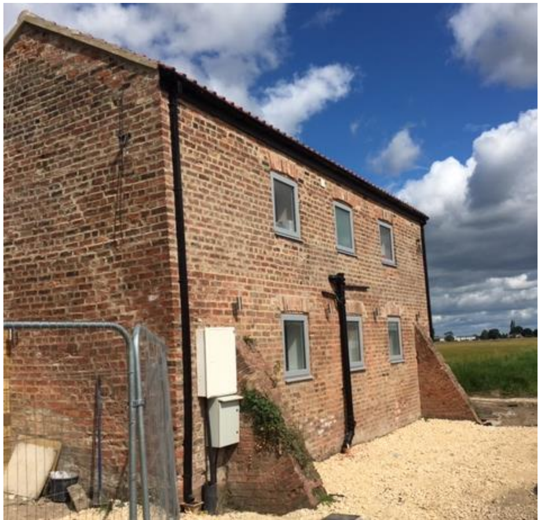
View of the east elevation
