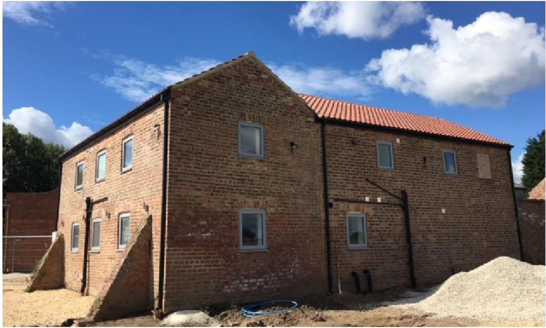
View of the north and east elevations from the highway
